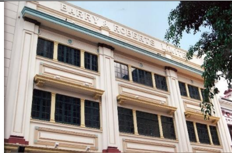
Barry & Roberts façade, Queen Street Mall Brisbane today
