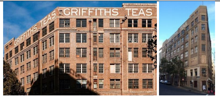
Griffiths Teas building Surry Hills Sydney
