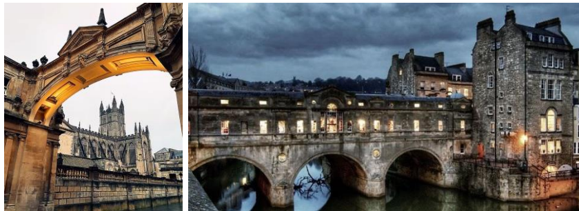
Pulteney Bridge, Bath – showing shops on the bridge
